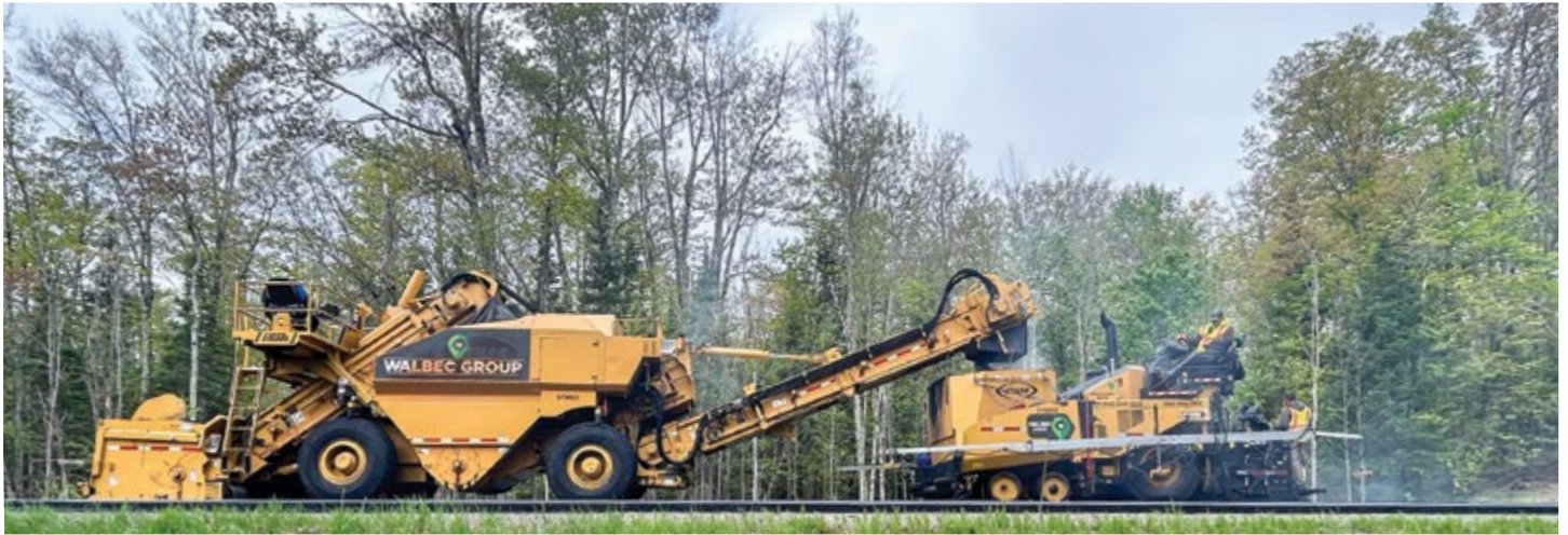
A Northeast Asphalt crew paving Highway B with a shuttle buggy to feed the paver for a continuous finish in Florence County,
